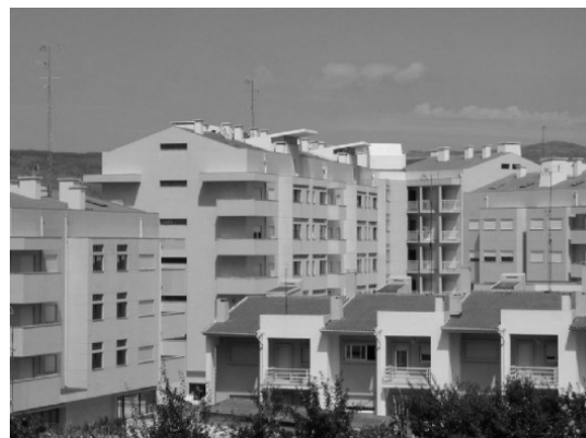
Figure 10: Typical tilted roofs.
