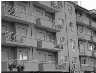
Figure 14 – Balconies and roller shutters used as shading devices.
