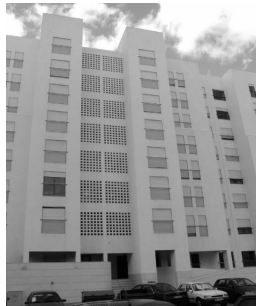
Figure 13 – Roller shutters used as shading devices.
