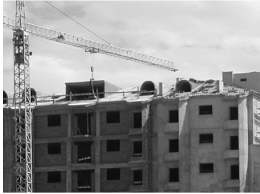
Figure 11 – Covering the roof slab with ceramic tiles.
