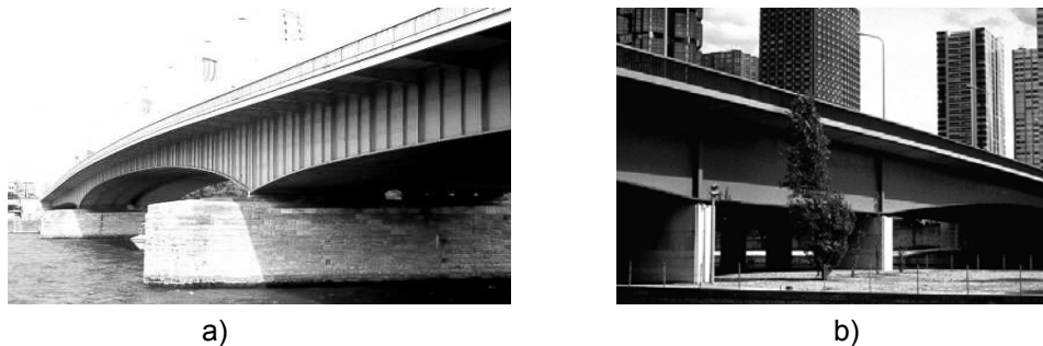
Figure 1 Tapered Plate Girder Bridge. a) Quai-Brücke Bridge, Zürich. b) Grenelle Bridge, Paris.[8]
