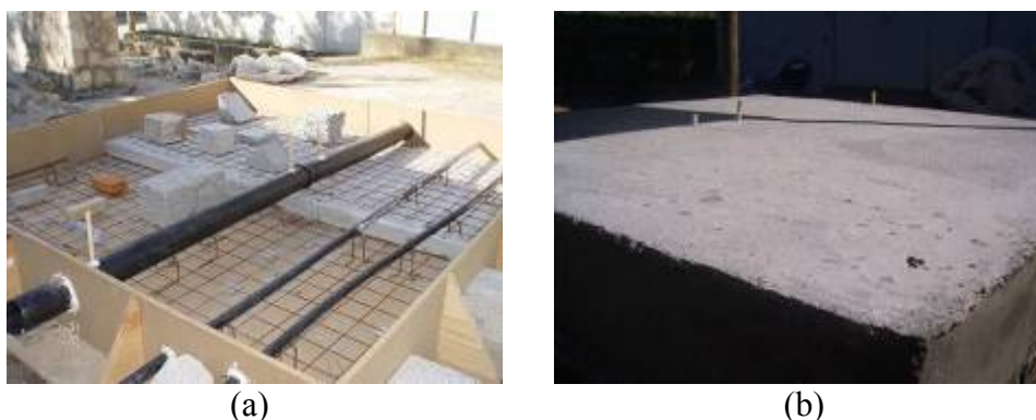
Fig. 1 General view of the concrete specimen. (a) Overview of the features and objects placed inside the specimen and (b) final view of the slab
