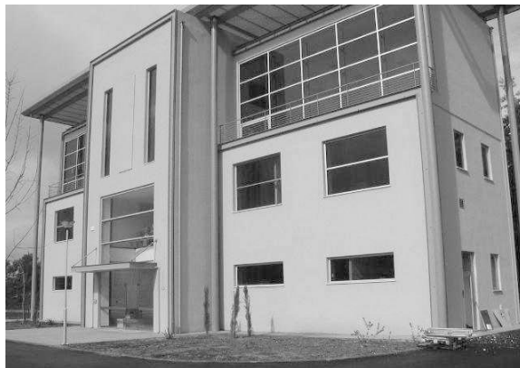
Figure 1. General view of the building where the MBT construction was implemented
