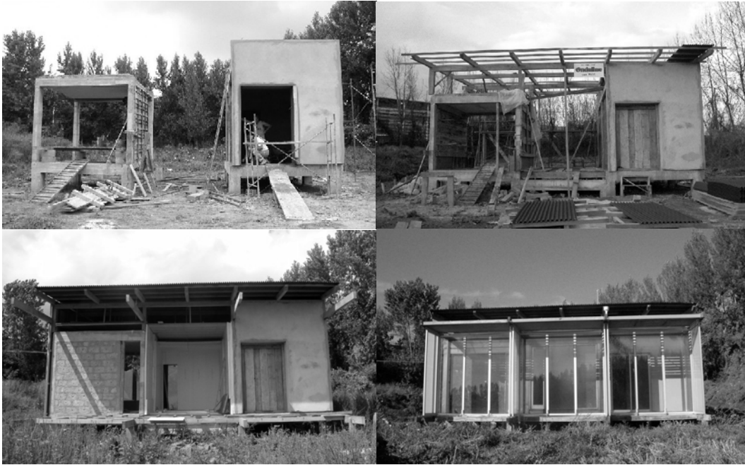
Fig. 7. Exterior views of the Building Test Cells Construction works
