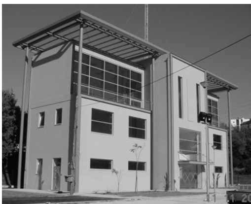
Figure 7. Front and lateral view of the building
