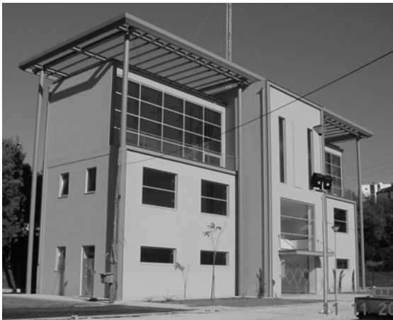
Figure 6. Front and lateral view of the building
