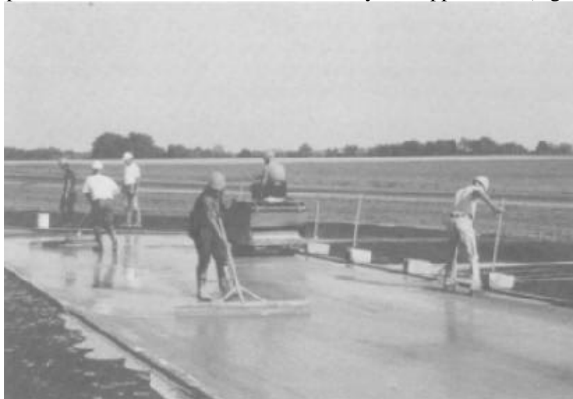
Figure 2 – Application of the cement grout on the porous bituminous layer
