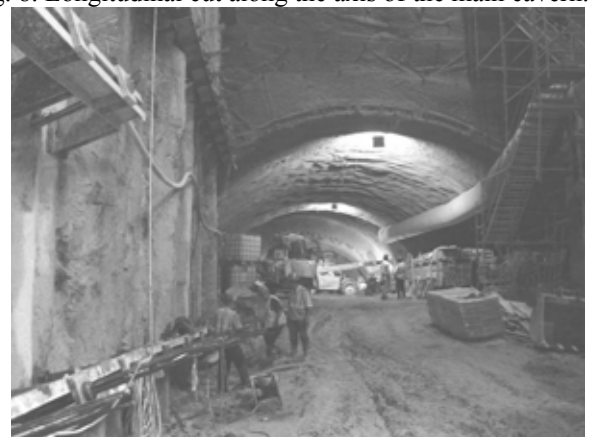
Fig. 9. Photo of the cavern in construction stage.
