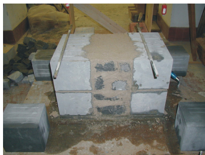
Figure 5.2 – Construction of the wallets.
