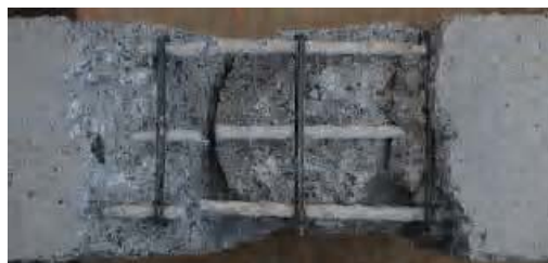
Figure 10 – Beam produced with braided reinforced composite rods after testing
