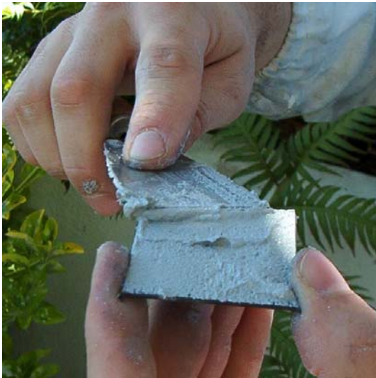
Fig. 4 – Application of epoxy on a CFRP plate.
