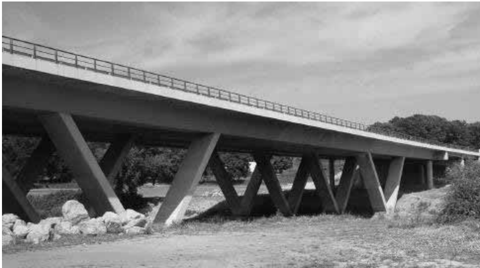
Figure 1. Bridge over the Ave River.
