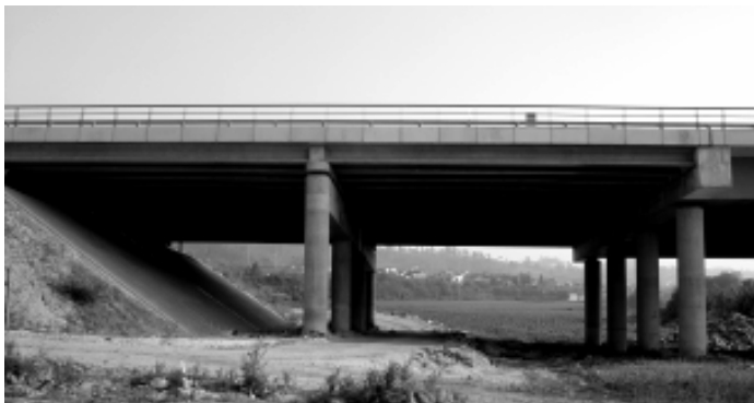
Figure 2. East access viaduct of the bridge over the Ave River.
