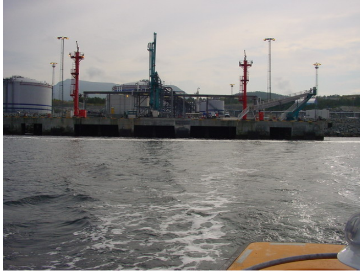
Figure 6.29 – Approach to Structure 3 from the fjord.
