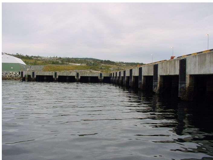
Figure 6.40 – View of Structure 4 from the fjord.
