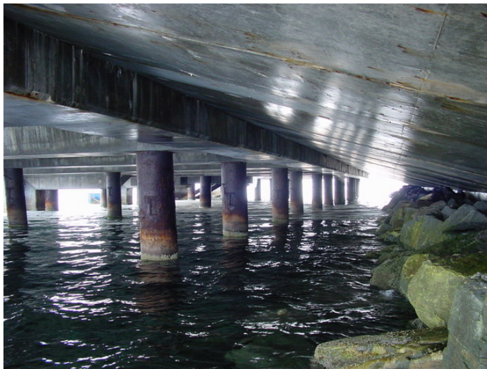
Figure 6.30 – View of the anchor slabs and beams under Structure 3.
