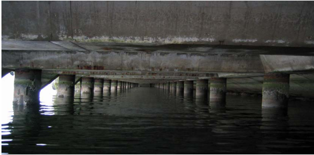
Figure 6.16 – View under the harbour structure.
