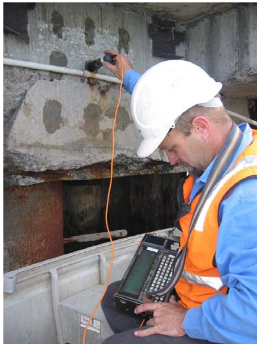
Figure 6.4 - Half-cell potential measurements being made on a wharf structure.
