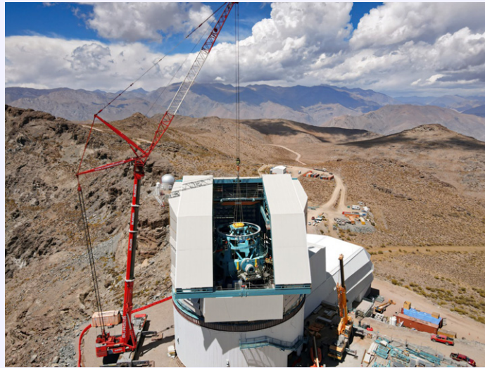
Construction at the Vera C. Rubin Observatory. Credit: ESA/Hubble, Rubin Observatory/NSF/AURA.
