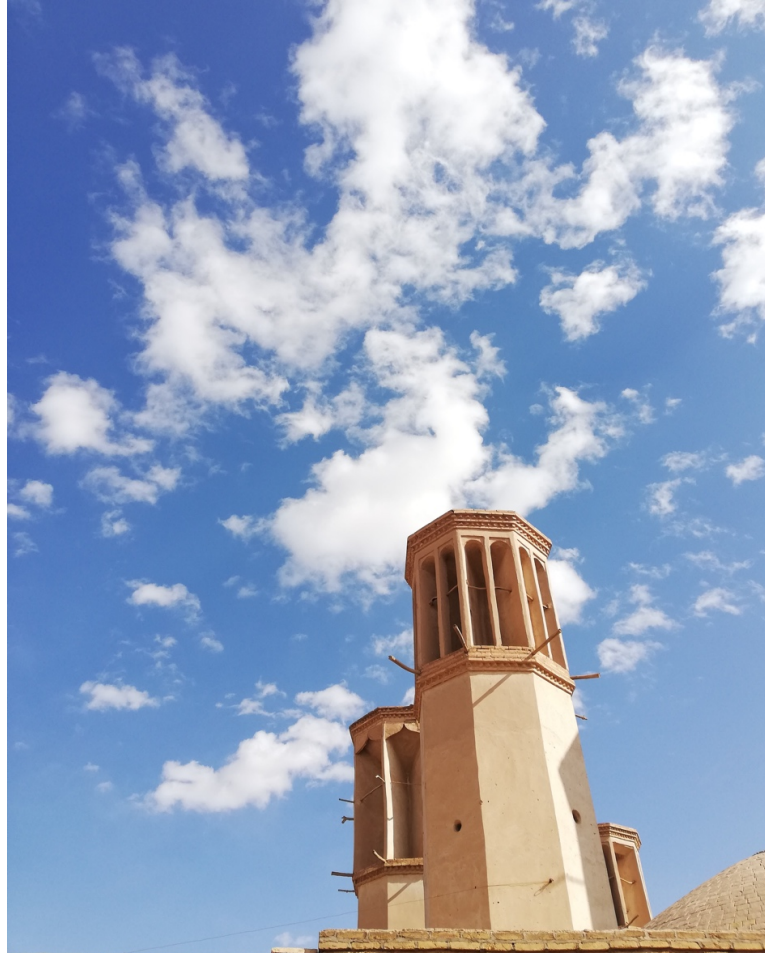
Figure 8.10: Windcatchers in the central Iranian city of Yazd. Photo from the personal collection of Mahsa Mojib.
