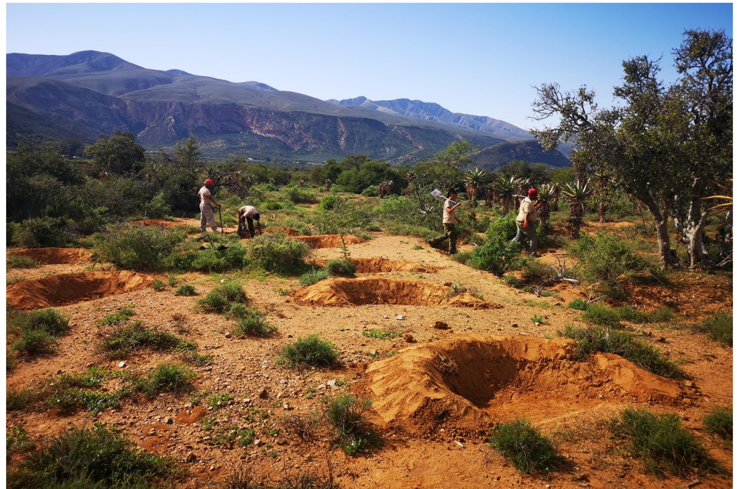
Figure 4. Constructing half-moon pits to capture runoff in degraded landscapes in the Baviaanskloof Hartland, South Africa (Source: Living Lands, 2020).
