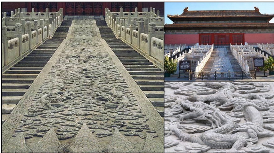
Figure 1.2: ‘The Large Stone Carving’ (left) is placed as a ramp flanked by stairs towards the Hall of Preserving Harmony, Baohedian (right top). The heaviest stone of the Forbidden City is 16 m by 3 m by 1.7 m with a weight of 200 tons [10]. It originally weighed roughly 300 tons; when it was re-hewn in 1761, its weight was reduced to about 200 tons. The chiselled ornamentalations on the stone include the dragon (right bottom), the symbol of celestial power. The pictures are from www.dpm.org.cn .
