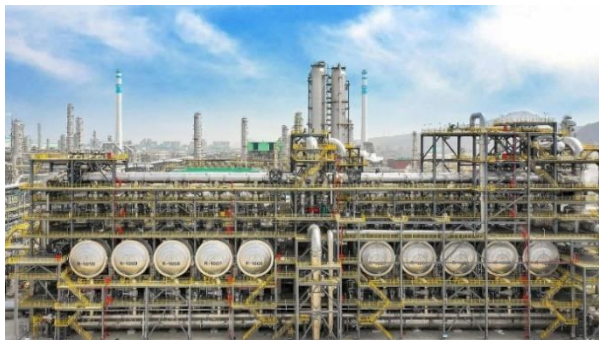
Figure 1.5. Propane and butane dehydrogenation plant of Hengli Petrochemical (Dalian, China) Refinery Co., Ltd using the CATOFIN catalyst. [64]
