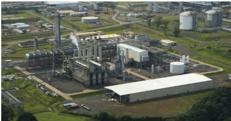
Figure 1: Methanol plant from Atlantic Methanol in West Africa that produces 1,000,000 metric tons of methanol per year. Photo from atlanticmethanol.com reproduced with permission.
