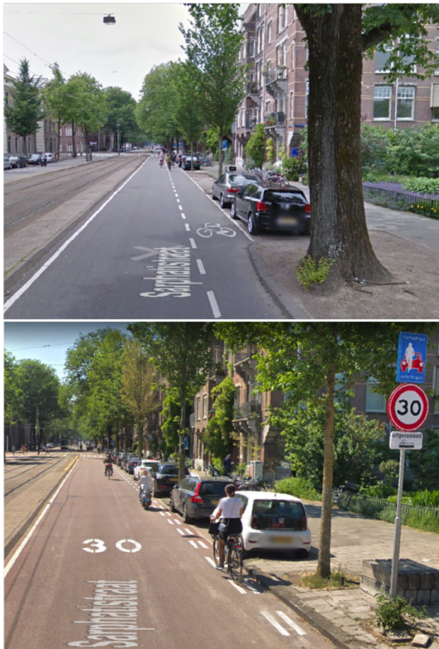
Figure 6.7 – Sarphatistraat before (above) and after (below) its redesign as a “bicycle street” (Source: Google Street View)
