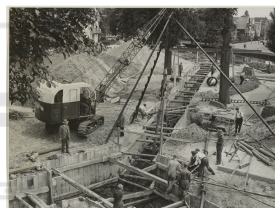
(c) Construction Site.
