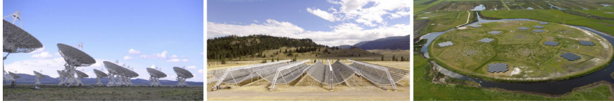
Fig. 9 Examples of radio interferometers used to search for FRBs (from left to right): the Jansky Very Large Array (JVLA) of 2725 m dishes in New Mexico, USA, the Canadian Hydrogen Intensity Mapping Experiment (CHIME) with four cylindrical paraboloids each 100 m long and 20 m in diameter in British Columbia, Canada, and the core of the Low-Frequency Array (LOFAR) of dipoles in the Netherlands
