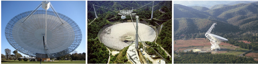
Fig. 8 Examples of single-dish radio telescopes used to search for FRBs (from left to right): the 64 m Parkes telescope in New South Wales, Australia, the 305 m Arecibo telescope in Puerto Rico, USA, and the 110 m Green Bank Telescope in West Virginia, USA
