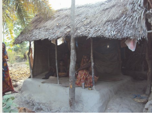
Image 4.5: house of an extreme poor family in Dacope
