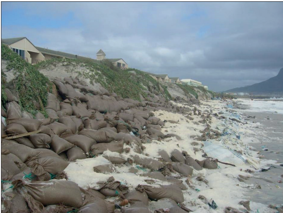
Figure 4.5: An example of how failed private interventions to protect property lead to a loss in the recreational, aesthetic and the tourism potential of beaches and the subsequent transfer of risk to the broader public
