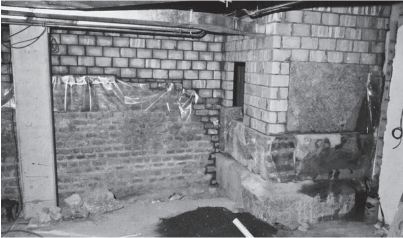
Fig. 5. The inner side of the west wall and gate of the late-Roman fortress during the restoration and reconstruction activities in 1987.
