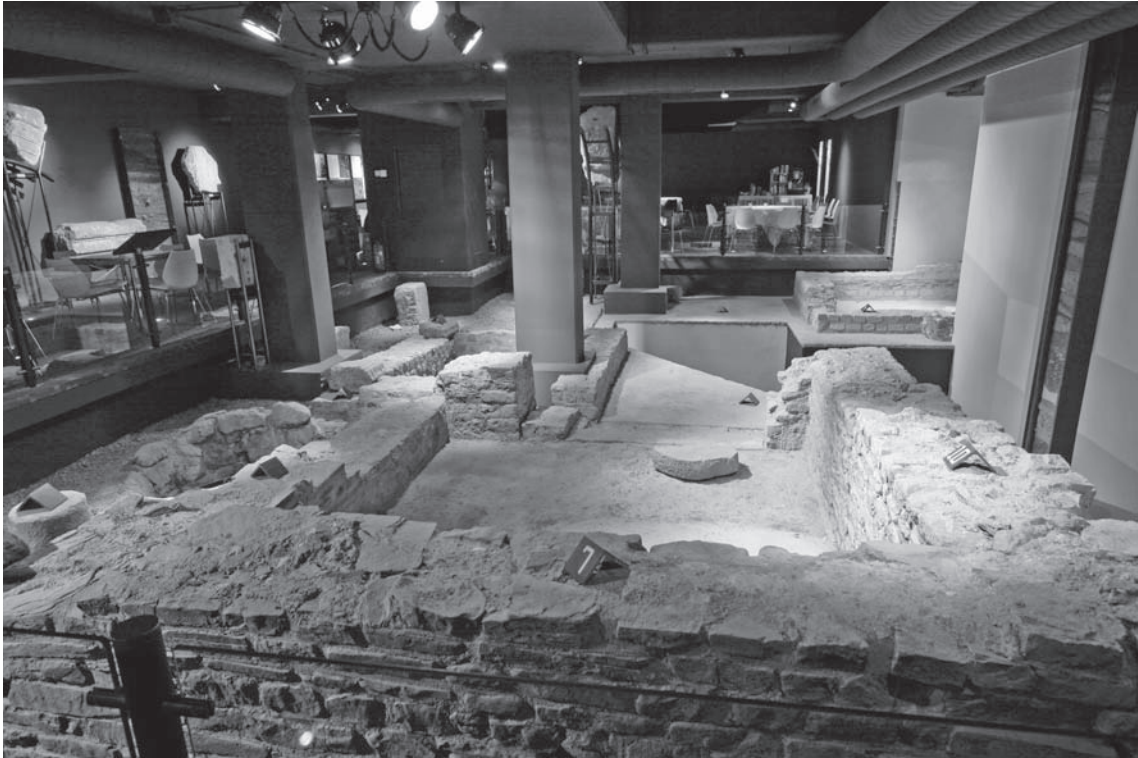
Fig. 10. View from the west across the consolidated and partly reconstructed excavation in 2007. Nearest to the viewer is the west wall of the sanctuary enclosure with renewed joints in the masonry.
