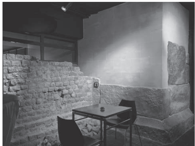
Fig. 7. The inner side of the west wall and west gate of the late-Roman fortress after the renovation of the Hotel Derlon Museum Cellar in 2007. The reconstructed section of the west wall of the fortress has been removed to give access to the new hotel bar.
