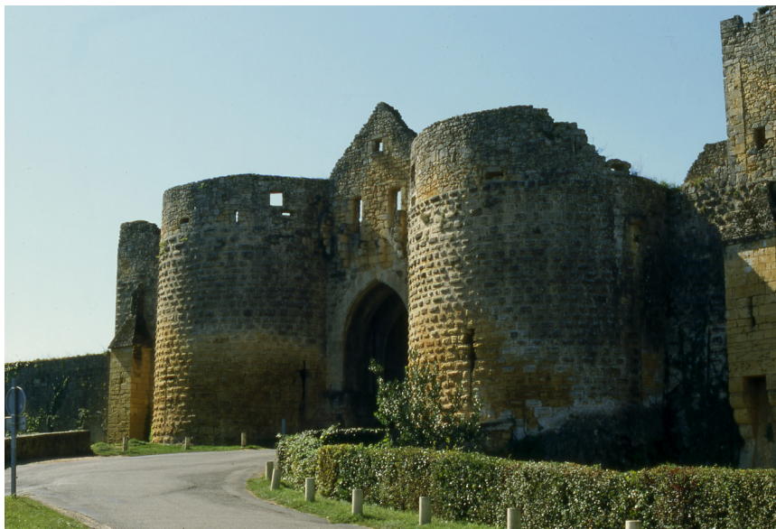
fig. 2.16: Eastern gate of Domme, from the northeast. The fortifications of Domme, which was founded in 1281-83, were built in the early 14 th century.
