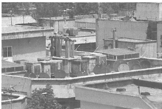
Figure 7.1 Common urban residential rooftops in Iran (photograph by kamshots [Kamyar Adl]).
