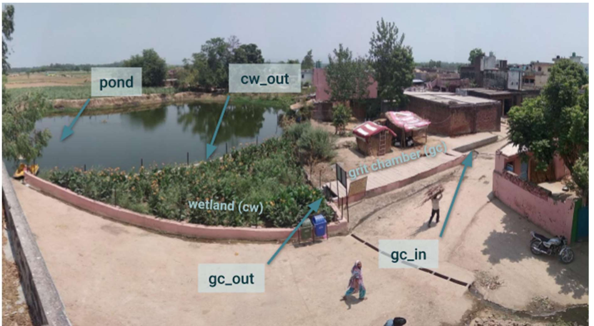
Figure 3.1 - Sampling locations at Ibrahimipur wetland. The codes in this figure are also used in charts in following chapters. gc_in: entrance to the grit chamber, gc_out: exit of the grit chamber, inlet to the wetland, cw_out: exit of the wetland into the pond.
