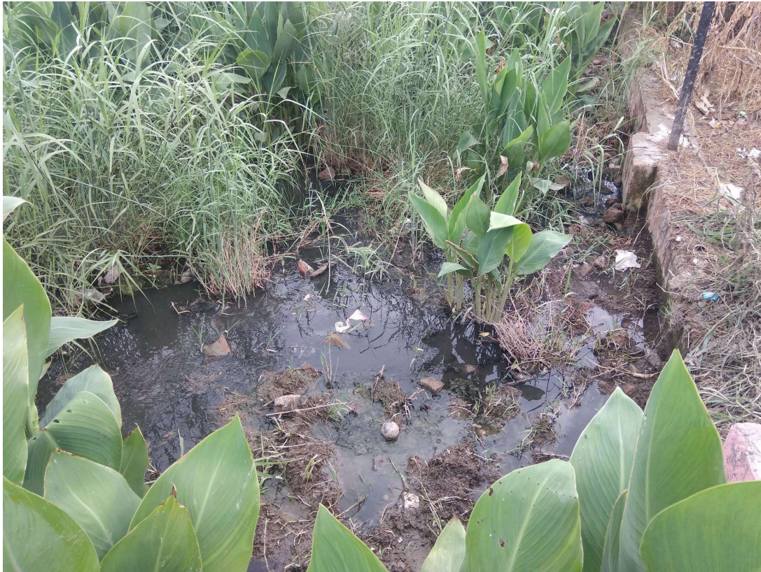
Figure 6.7 - Clogging and surface flow around canna and reeds at Ibrahimpur. When first constructed, this wetland was clean bricks and stones, with no mud. Photograph by the author, 2020.
