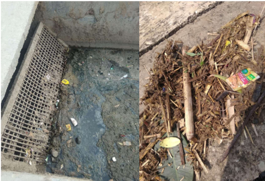
Figure 6.10 - Ibrahimpur grit screen clogging, with dried solids on right showing the predominance of straw. Photograph by the author, 2020.
