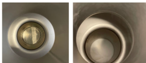
Figure 13: Inside the twin axis cavity #1 after the second coating.
