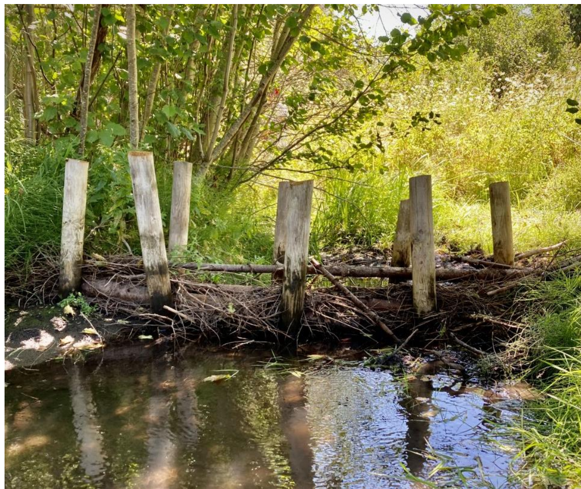
Example of a BDA used as a restoration technique to reduce incision and head cuts in Fish Creek, Montana
