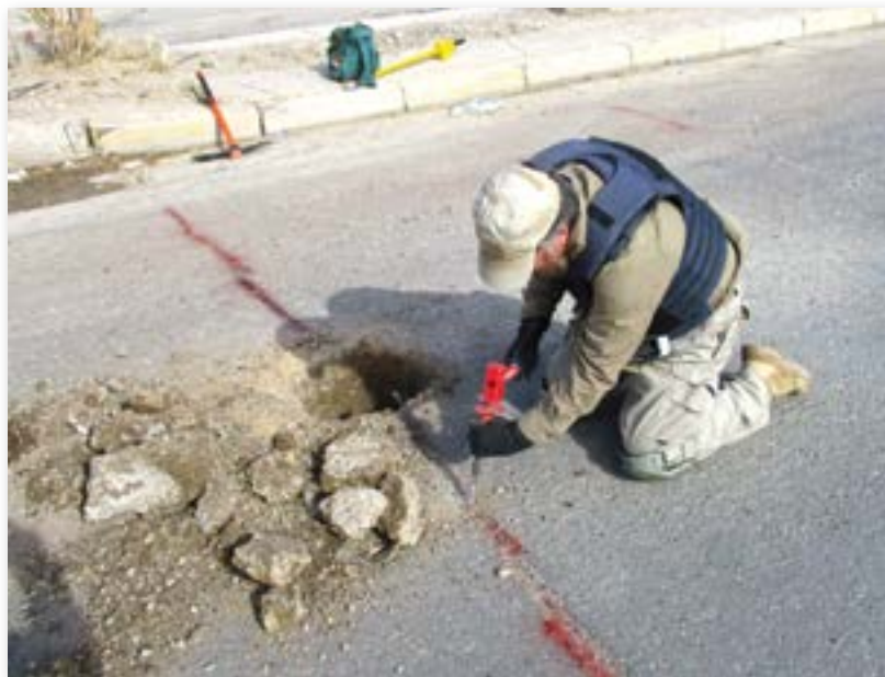
Image 14. Cautiously chiseling detonating cord out of Highway 10 in Fallujah, Iraq.
