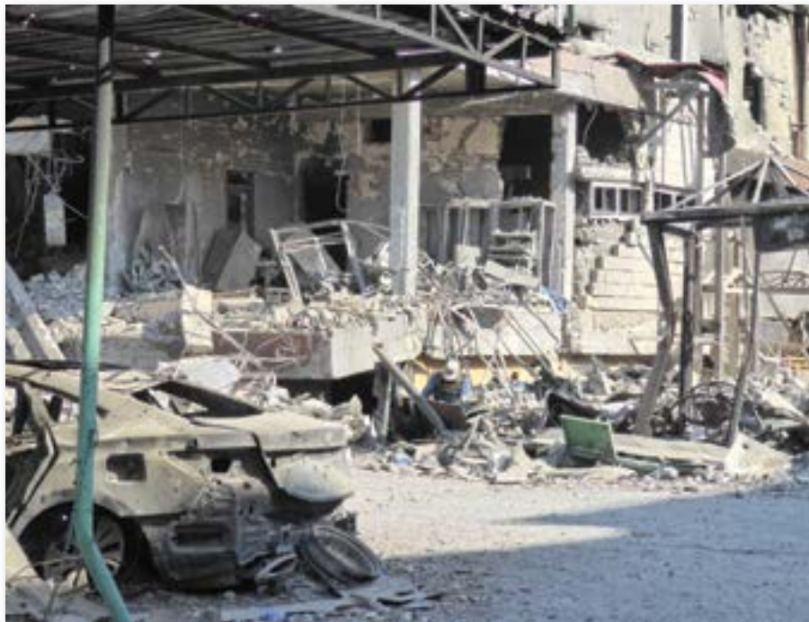
Image 3. Some clearance locations present special hazards (i.e., mixture of ordnance and IEDs, falling debris, unstable structures, etc.).
