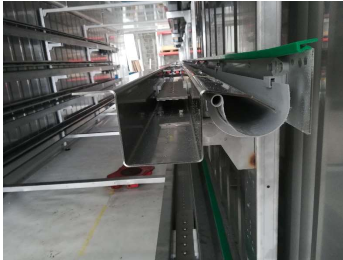
Figure 16 - Close up on the Tacker rail and irrigation gutter
