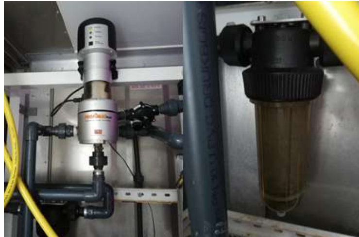
Figure 17 - On the left: Automatic Filter; On the right: Basic filter for the backwash
