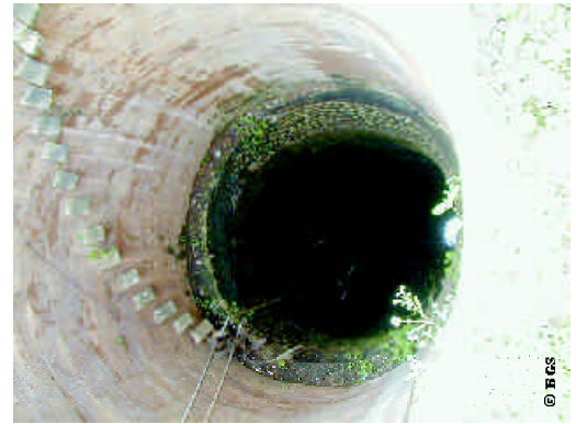
A dug well deepened as groundwater levels decline
