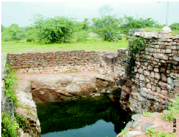
A well located in a pocket of shallow weathered hard-rock, down-gradient of a checkdam, Coimbatore District
