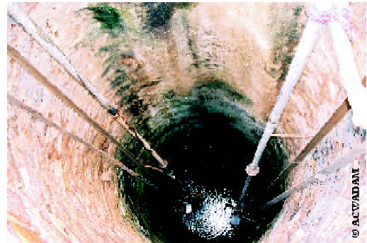
Sharing out of inherited land, and in turn access to water, can mean competition even within wells. Here two pump sets are relocated within a shared dugwell
