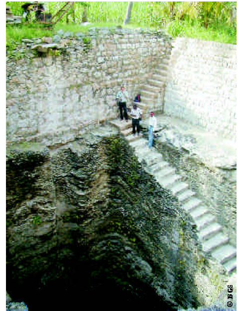
A large diameter well, Coimbatore District, deepened due to declining groundwater levels
