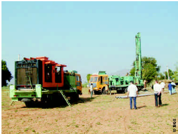
A group of farmers have joined resources to drill a borehole in the Satlasana area of Gujarat. Three previous attempts had found little water.
