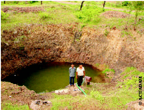
A Pani Panchayat well, where water levels have dropped due to groundwater overabstraction in surrounding areas
