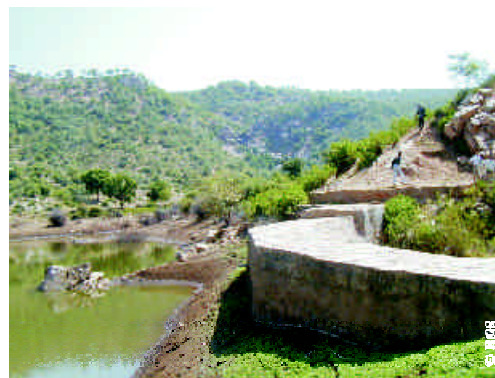
A checkdam in a narrow steep-sided valley in the Arwari River Basin
