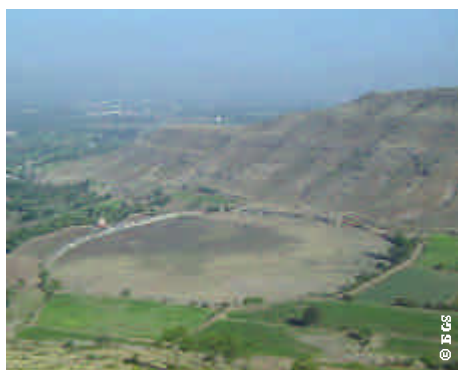
An old tank near Pune now almost totally silted-up
