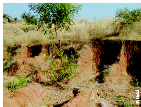
Excavation to provide storage upstream of a check dam. Households are paid by the volume of material removed: small earth walls show the boundaries between where different households have been digging.
