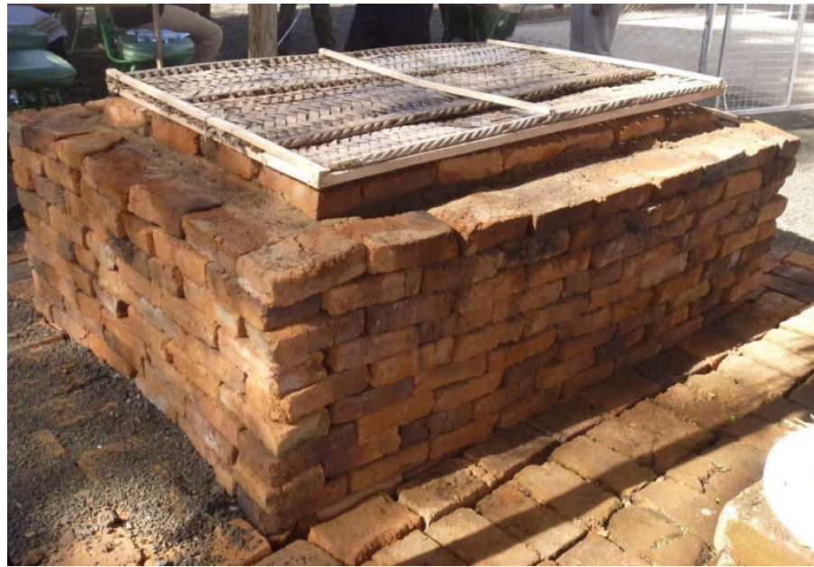
Figure 2. Zero-Energy Cooling Chamber for storage of fresh fruits and vegetables in Tanzania [53].
