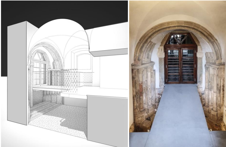
Fig. 12. Architectural design of how the portal is to be exposed with the use of a footbridge leading to the church
