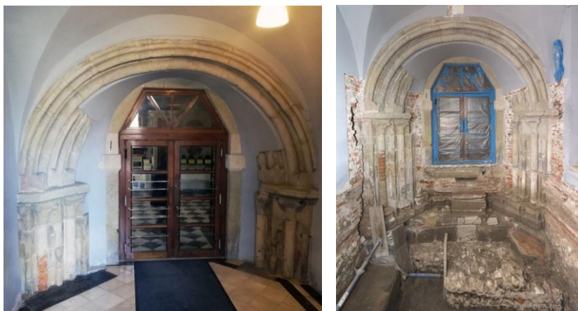
Fig. 1. The condition of the portal before the works in 2019 and after the completion of archaeological research in 2020
