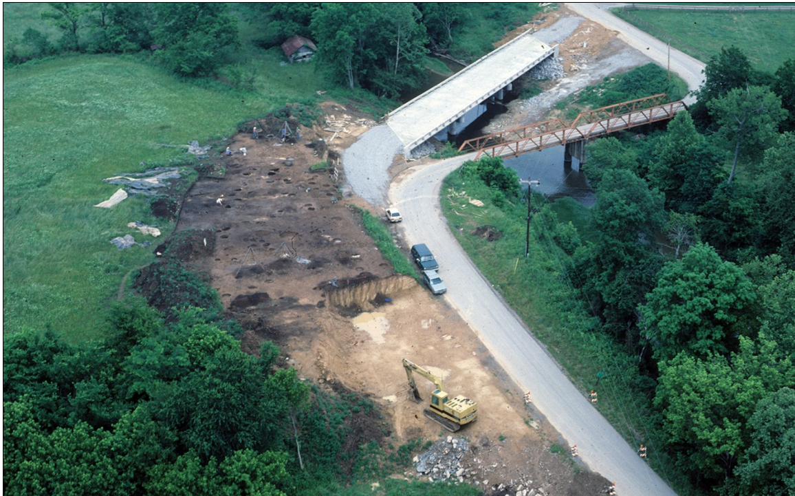
Figure 3. Aerial photo showing data recovery excavations and road construction.
