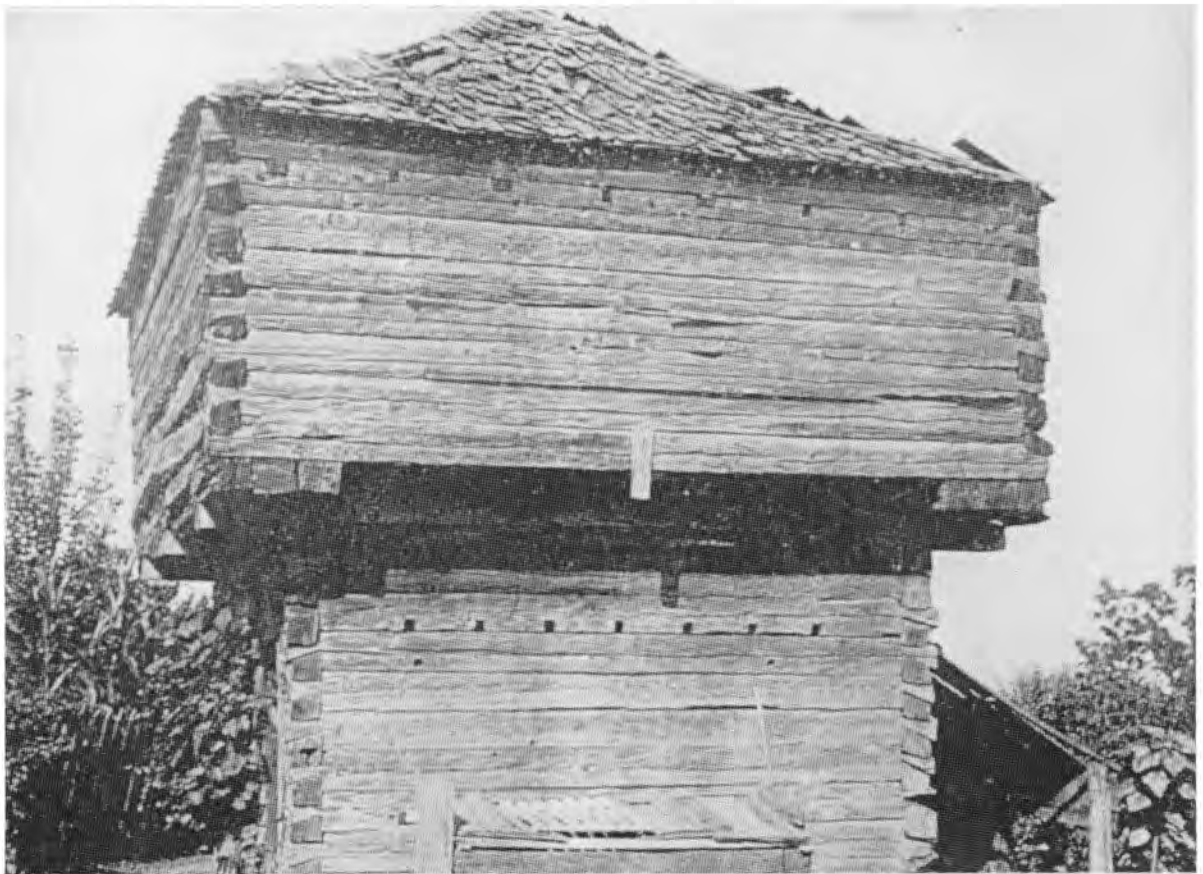
Figure 37. Pre-1922-relocation photographs of the Fort Marr Blockhouse (upper from Penelope Allen Papers, CC; lower from Cline 1942:Plate 39).
