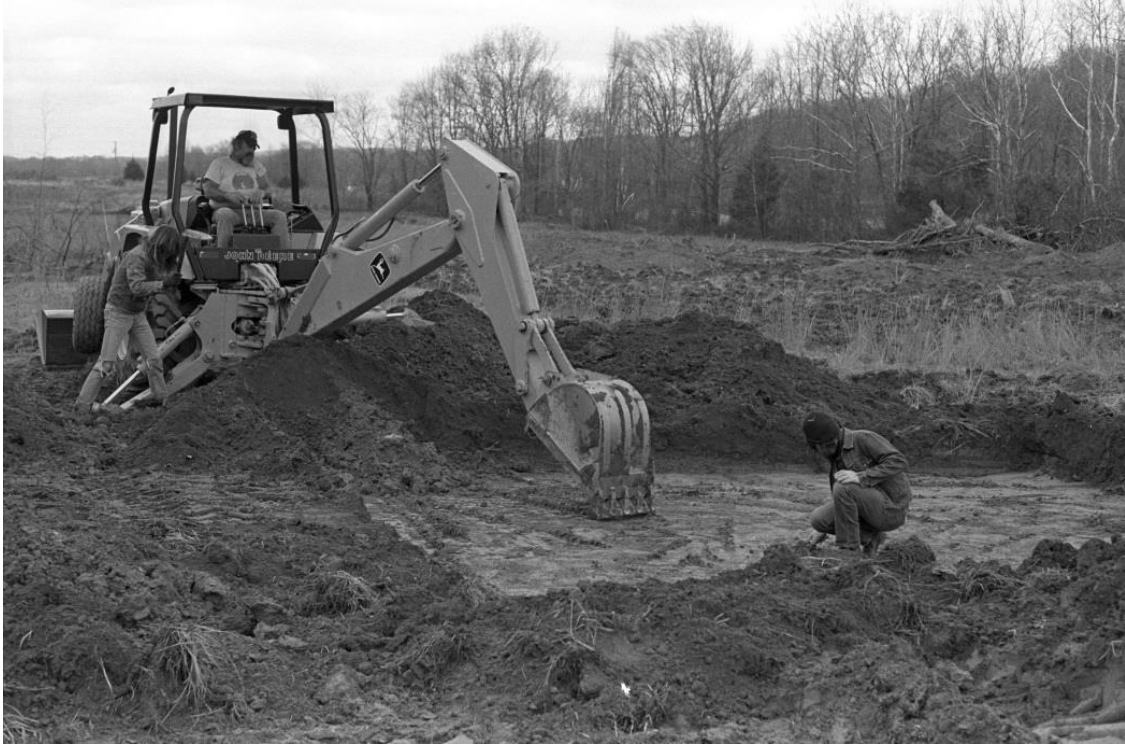
Figure 8. Crew during excavation of Strip Block 2 at site 40PM34.
