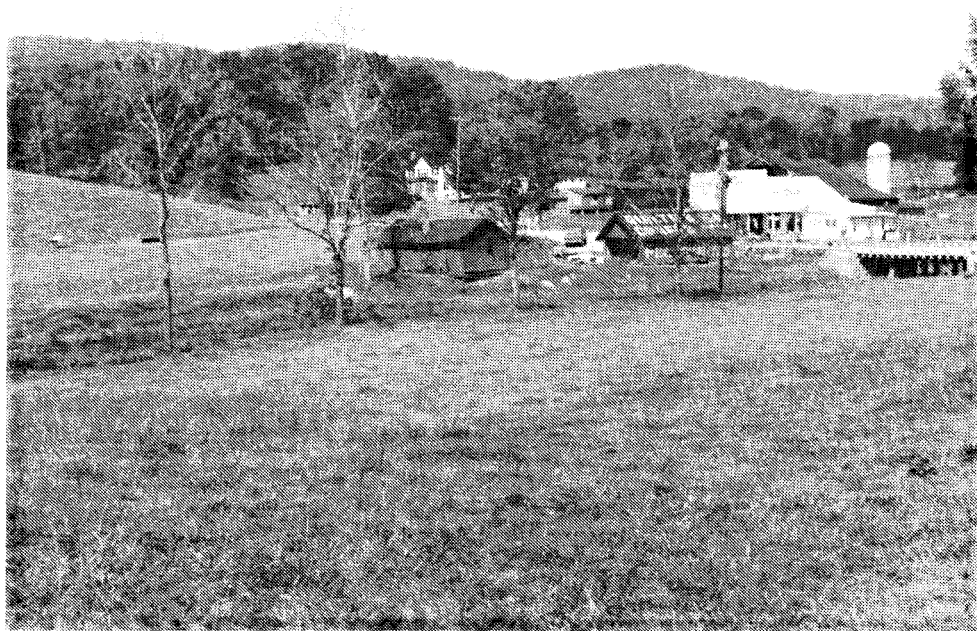
Figure 22. Cattle Weighing Barn, Blacksmith Shop, Forbus General Store, and Manager's House. Looking West Across the Site.
