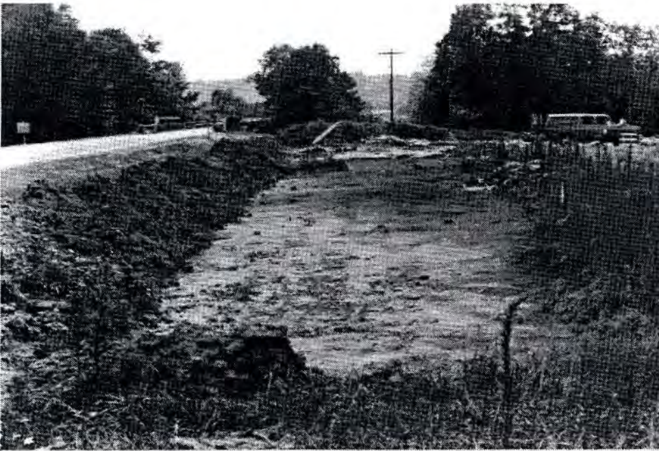
Figure 7. Power Unit 1 and Power Unit 2. Unit 1 (Top) Looking East and Unit 2 (Bottom) Looking South.
