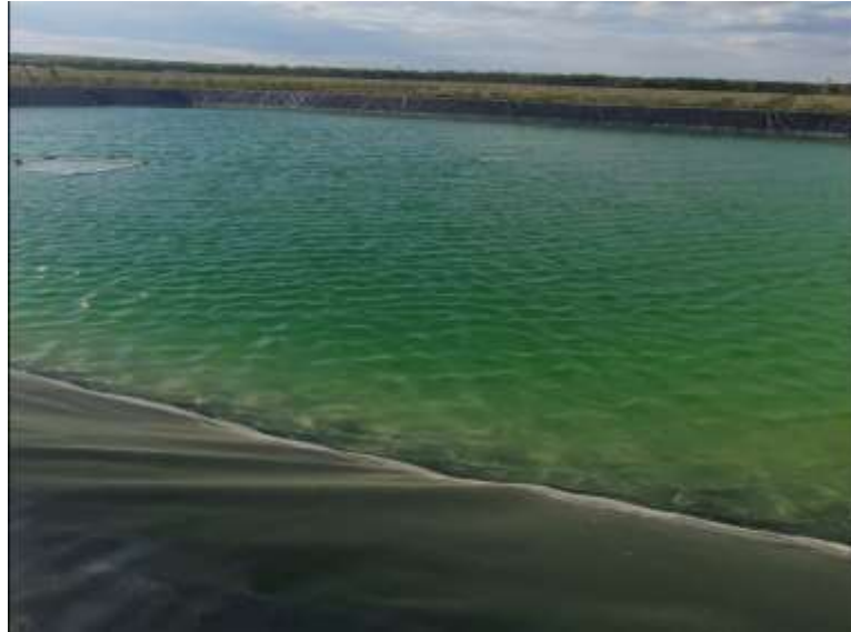
Figure 1 Storage and distribution tank
