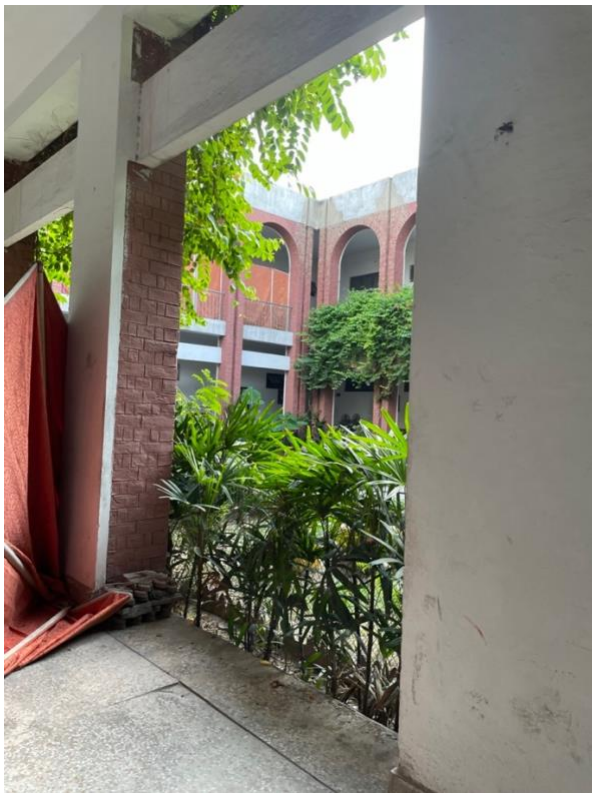
Figure 7: Corridors at Dharampura College
