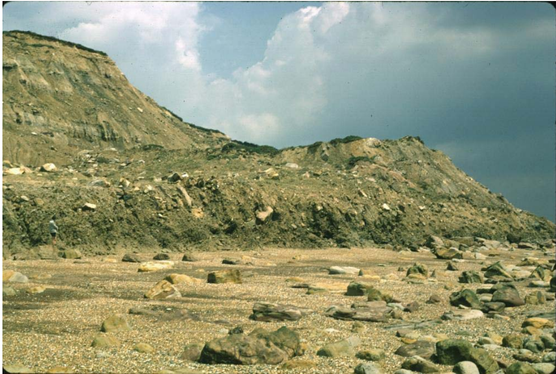
A11341: Landslip, LeeNess
