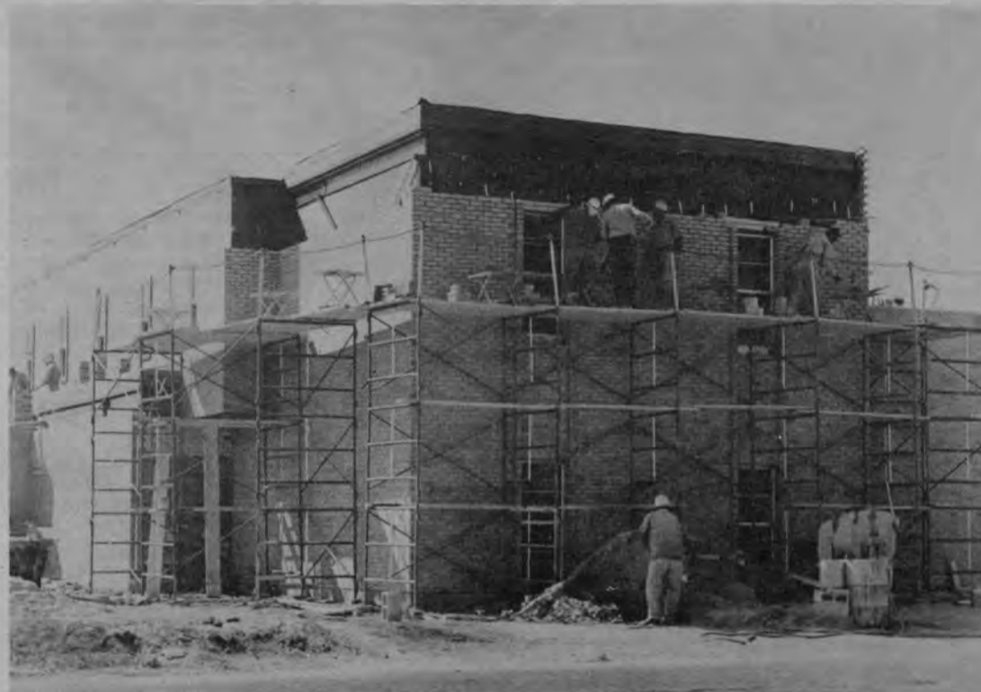
Work Proceeding On New Center
