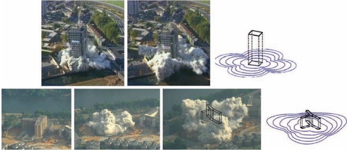
Fig. 1 Field observations of a non-circular gravity current. Aerial views of ( top ) a building of square cross section and ( bottom ) a T-shaped building being demolished. The structure of the debris cloud is highly dependent on the building's shape. Observe that material very close to the center of the building moves farther out than material located at the building's extremities. The dynamics of the cloud is reasonably well captured by our proposed model, where the front location of the cloud is marked at equal instants of time as blue lines (color figure online)
