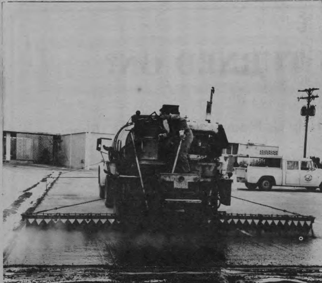
STATE HIGHWAY DEPARTMENT workers in the above photo are spraying tar on the library parking lot. According to Louis S. DeVries, maintenance director, the department plan is to resurface all the parking lots and driveways on campus. He said, "It will take care of everything we've got."
