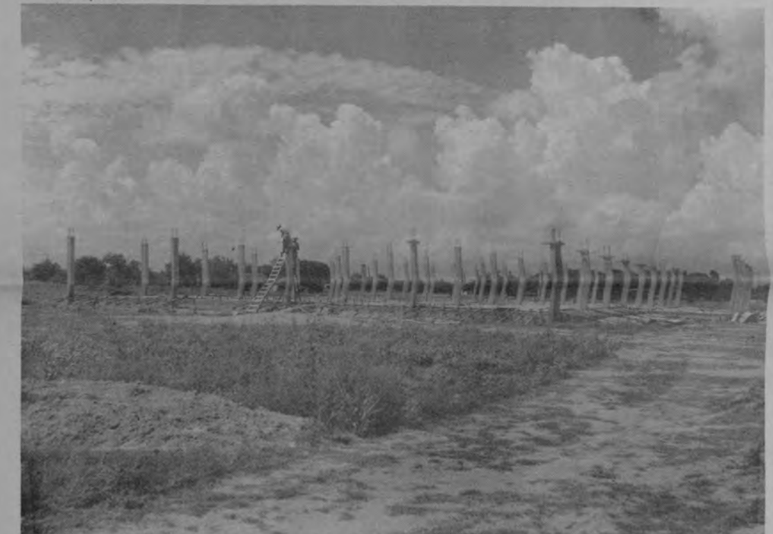
SKYLINE begins to rise on PAC's West Campus.
