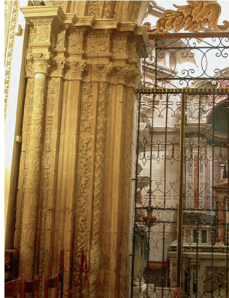
Fig. 13. Modica. Confrati chapel in the church of S. Maria di Betlem in Modica, detail of the entrance arch.
