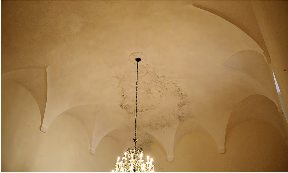
Fig. 24. Palermo. Villa Gonzaga (now the church of Santa Maria di Monserrato or delle Croci), detail of one of the original vaults.
