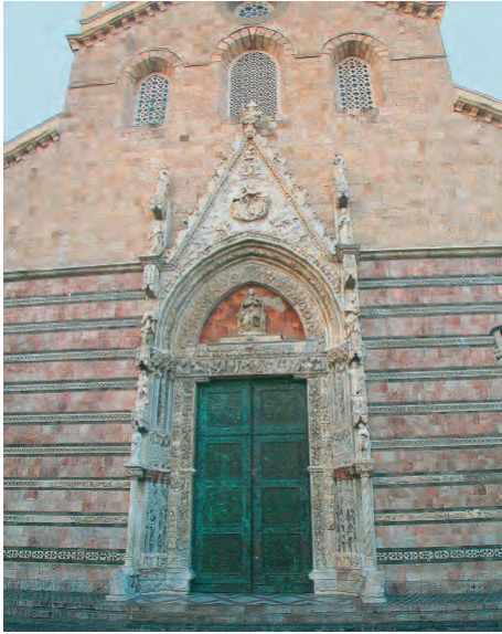
Fig. 28. Messina. Cathedral, detail of the façade with the multi-colored coating on the first order.
