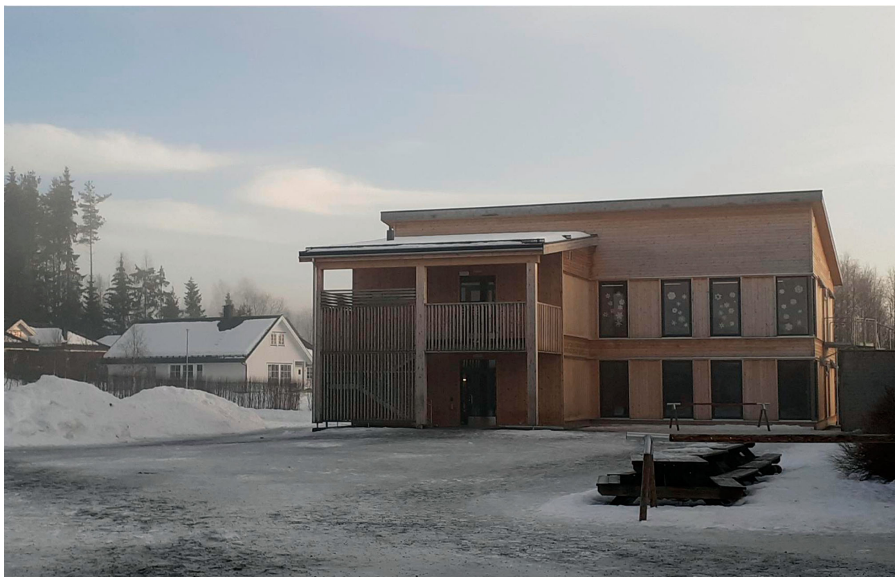
Figure 2. View of north façade January 2020. Classrooms 107 and 207 are located on the right-hand side of the building.
